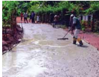
Provided financial assistance to concrete a rural road in Attanagalla
